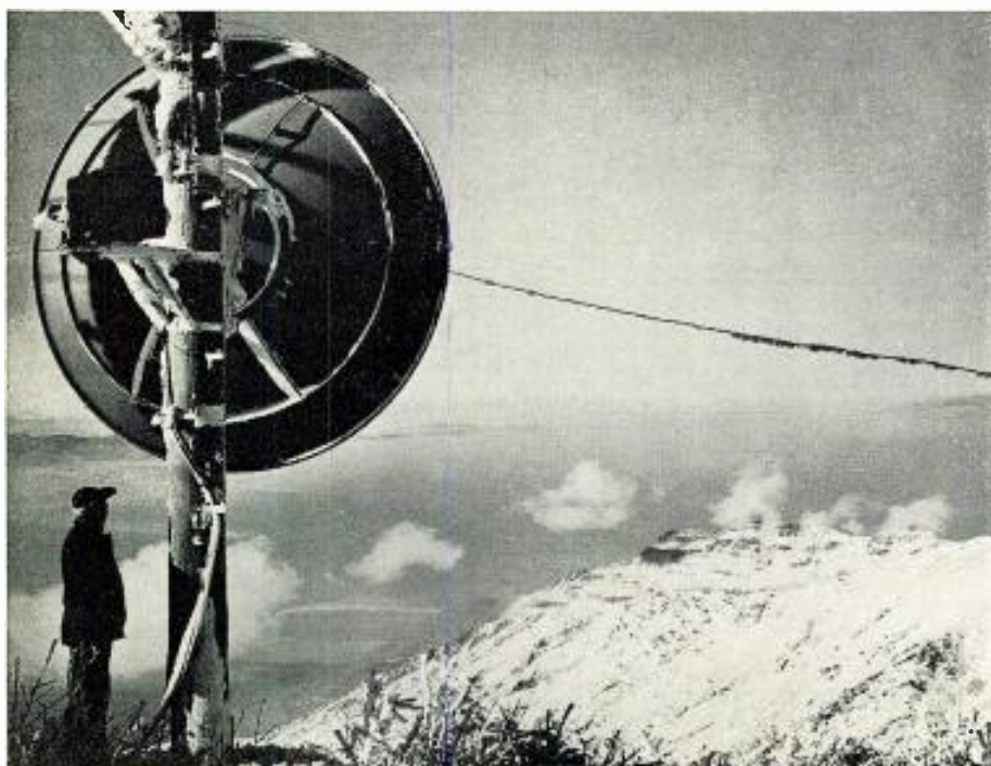
Fig. 1. Television microwave transmitted antenna installation.
